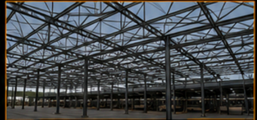
ROOF TRUSSES & PURLINS
