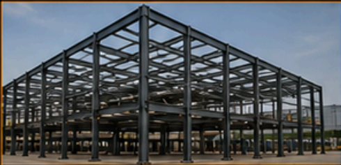
STRUCTURAL STEEL FRAME
